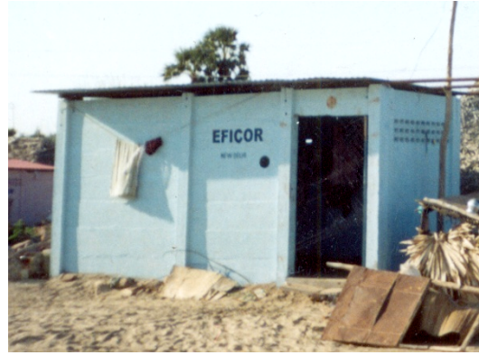
Fig.2. A Small Sized Temporary Shelter Without Adequate Provision for Light and Ventilation.
