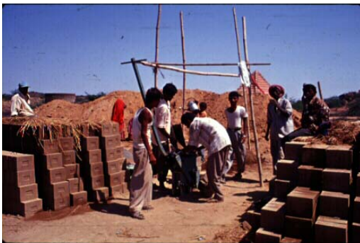
Figure: Compressed soil blocks used by Abhiyan for reconstruction
