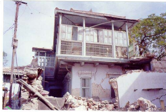
Figure: Some traditional constructions in wood and masonry survived due to special construction techniques – in Anjar.
