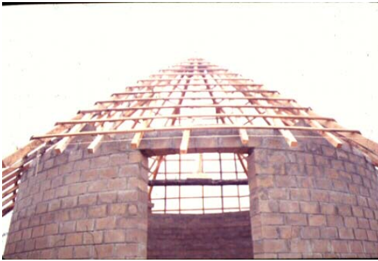
Figure: Bhungas (traditional housing form) reconstructed using compressed soil blocks by Abhiyan
