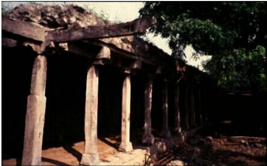
Figure Above: Traditional Malwad construction in wood withstood the impact of earthquake quite effectively.
